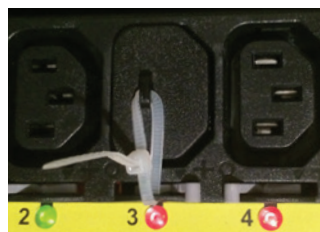
Cap secures in place with cable tie
